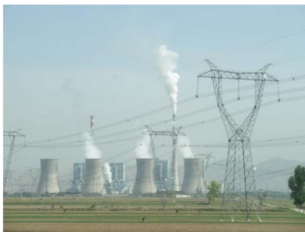
Figure 7.25 Tremendous amounts of electric power are generated by coal-fired power plants such as this one in China, but an even larger amount of power goes into heat transfer to the surroundings. The large cooling towers here are needed to transfer heat as rapidly as it is produced. The transfer of heat is not unique to coal plants but is an unavoidable consequence of generating electric power from any fuel—nuclear, coal, oil, natural gas, or the like. (credit: Kleinolive, Wikimedia Commons)
